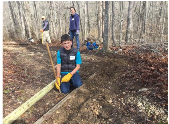
Star Scout Laiten Burnelle and mom Jennifer Burnelle installed water bar
