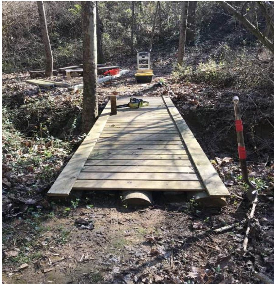
2 nd Trail bridge needing handrails
