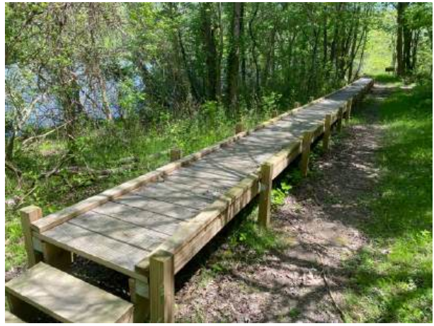
Completed 120-foot boardwalk at Pot Point in low-lying area
